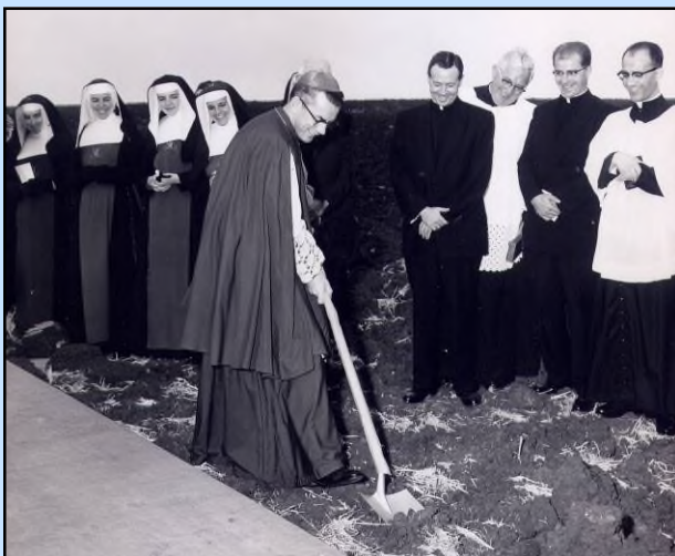
Ground Breaking for Mary & Joseph Retreat Center
